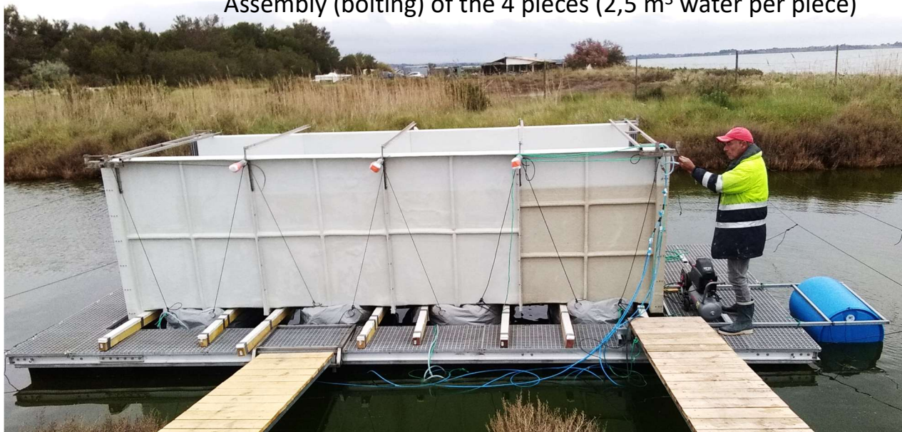
Assembly (bolting) of the 4 pieces (2,5 m 3 water per piece)
